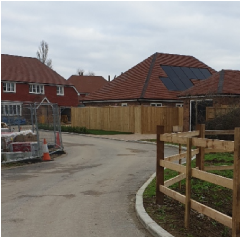
Figure 8 Recently consented fence on Jemmett Development
